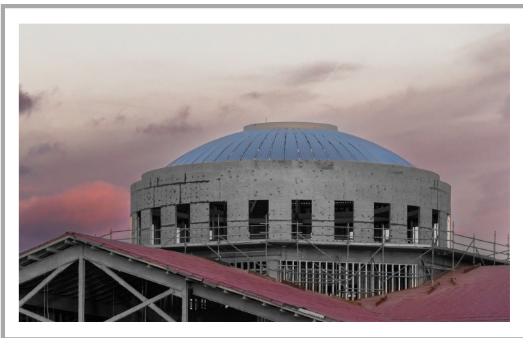
A view of the State House in progress from December 2025.
